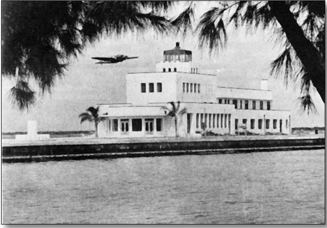
The administration building at Peter O. Knight Airport, which was built by the WPA on Davis Islands in Tampa.
